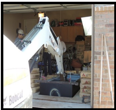
Shelter Being Installed
